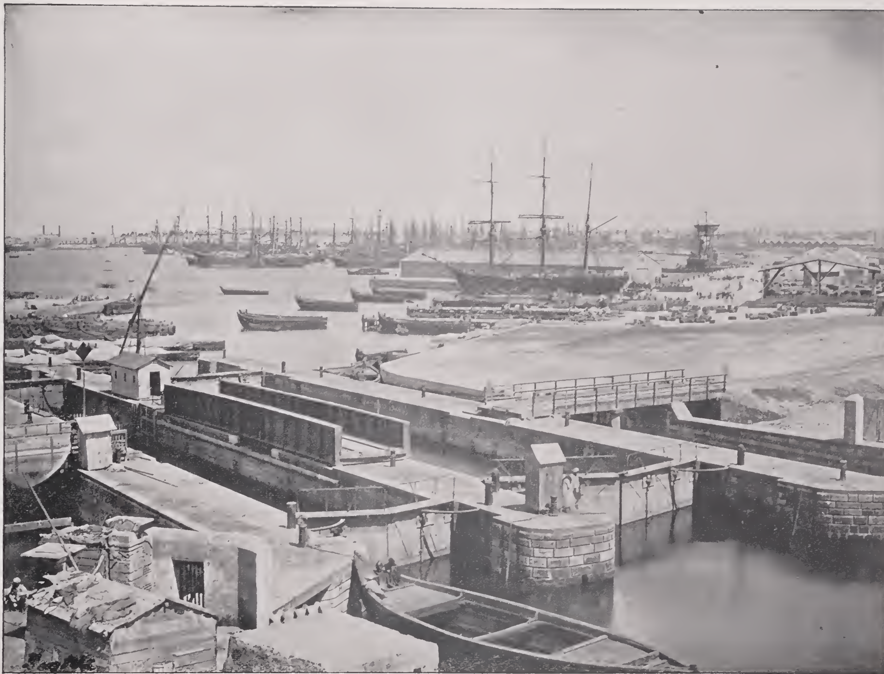
HARBOR, ALEXANDRIA, EGYPT.—The perfectly flat coast of Egypt, and even Alexandria itself, are not visible to the steam-boat passenger until very shortly before the vessel enters the harbor. The latter consists of an outer breakwater, forming an obtuse angle nearly two miles in length. A second pier, nearly a mile in length, protects an inner harbor covering nearly five hundred acres of water, twenty-seven feet deep. No fewer than thirty thousand artificial blocks, weighing twenty tons each, and two million tons of natural blocks of stone were used in the construction of these magnificent harbor works.
